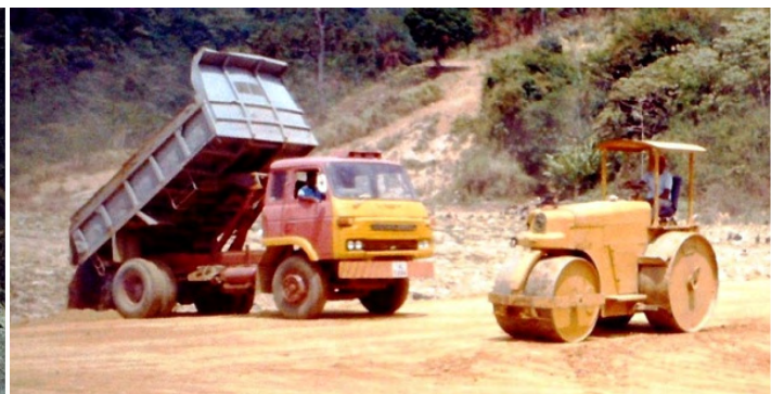
Photo B4.20 Road roller used to build a site road
