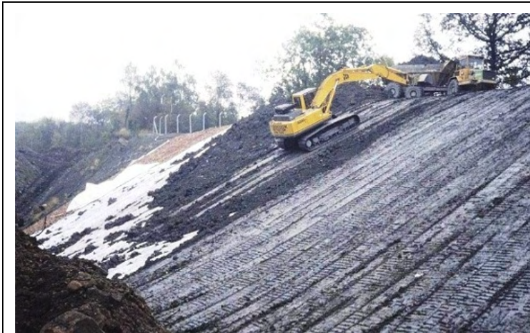
Photo C4.1 Lining the side of a landfill
