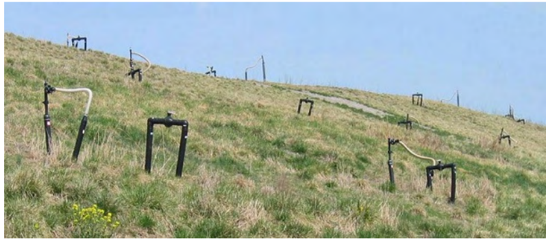
↑ b) Connected gas wells on a completed section of a large landfill
