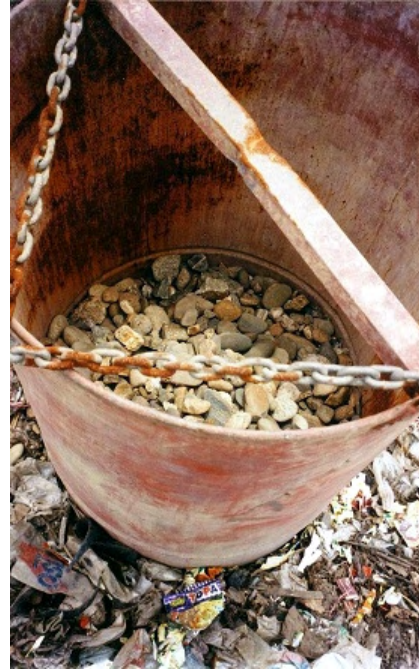
➤ b) Stones are placed in the casing to approximately the same level as the waste
