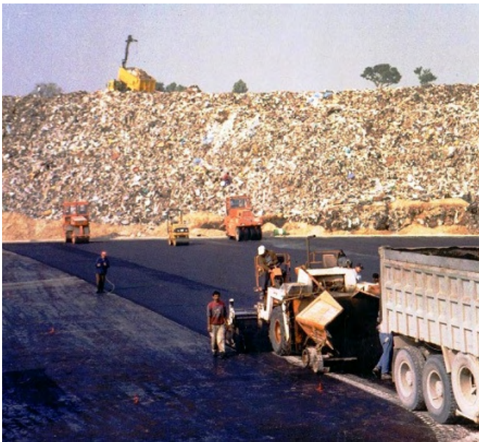
b) The asphalt is laid on the base (Note the waste piled up on the other part of the site)
