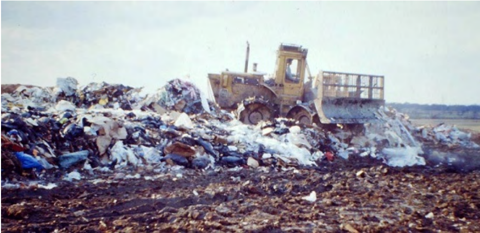
Photo C4.3 A landfill compactor at the working face, moving up and down the slope to compact the waste.
