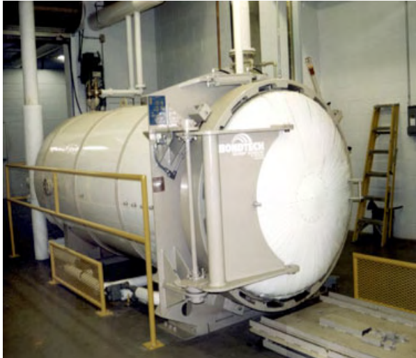
Photo B3.3 Autoclave for treating infectious waste
