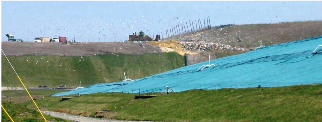
Photo B4.13 Temporary impermeable cover.
