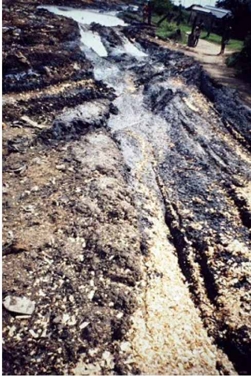
➤ a) If the access to the unloading area of the dump is like this, the vehicles bringing waste will experience many problems
