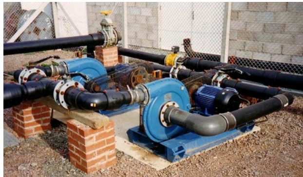
↗ c) Vacuum pumps that draw the gas from the wells
