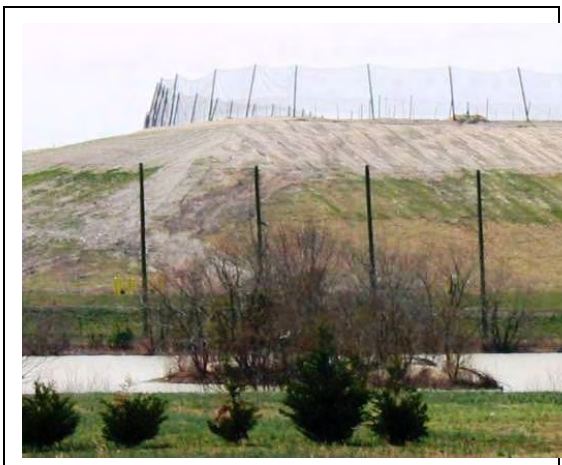
➤ c) The tall poles in the foreground and in the distance are supporting nets for catching litter
