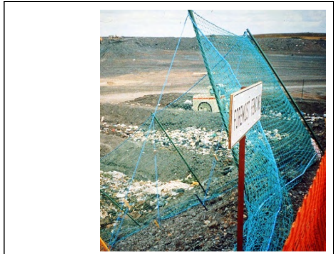
➤ b) These nets can be moved so that they are always downwind of working areas
