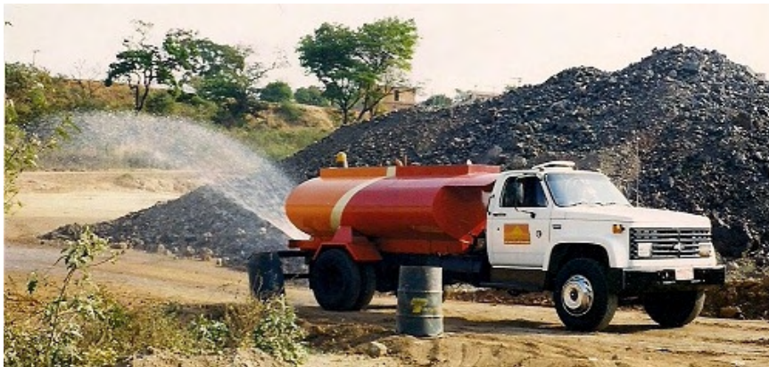
➤ c) Spraying to suppress dust
