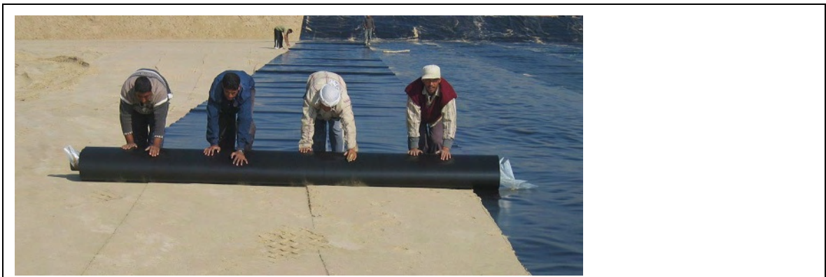
Photo B4.14 Construction of an impermeable liner.
