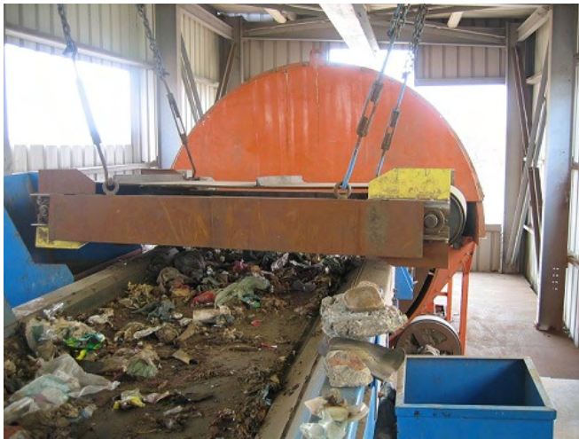
Photo B2.7 Magnet suspended over the end of a picking belt
