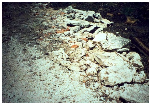
Photo B4.19 Broken concrete used to make a site road
