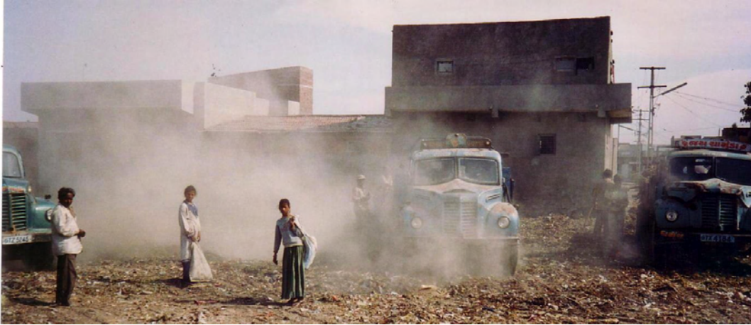
➤ a) Unloading waste creates a dust cloud
