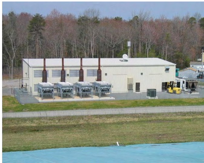
↗ e) Generating station on a large landfill, fuelled by landfill gas
