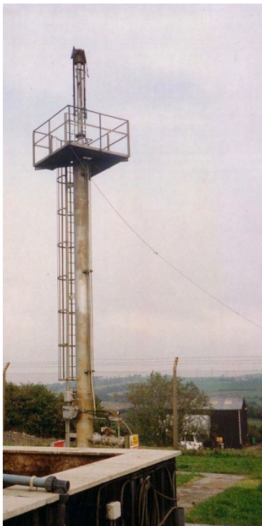
↑ a) Vertical gas wells that are raised as filling proceeds
