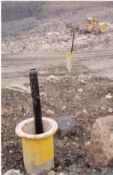
↑ a) Vertical gas wells that are raised as filling proceeds
