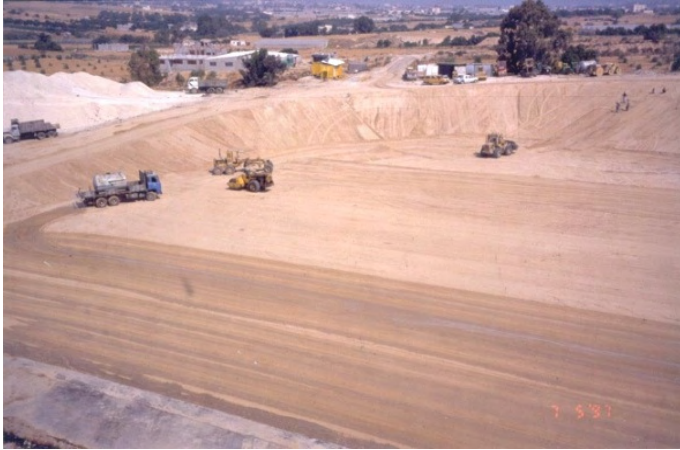
a) The site is prepared for the asphalt
