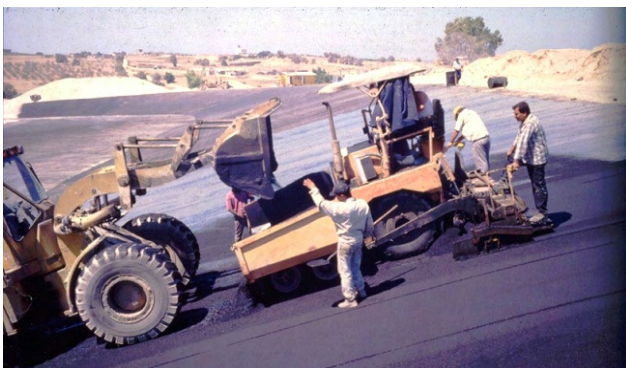
c) Laying the asphalt on the sides
